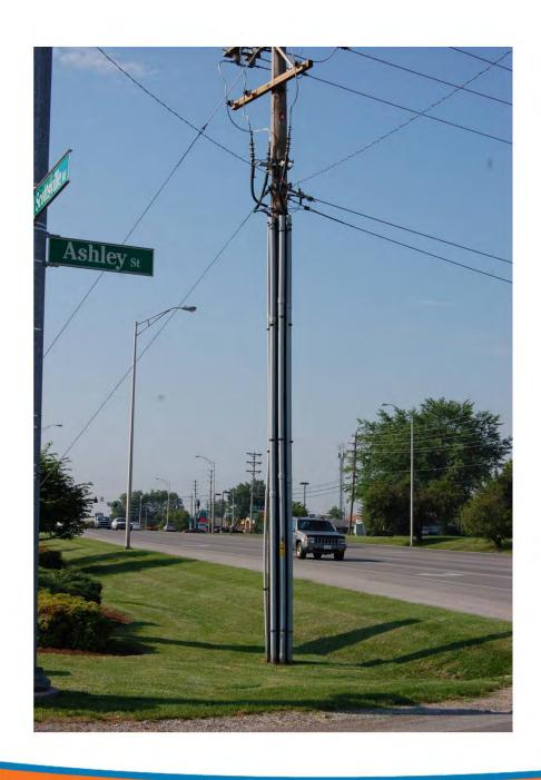
Overhead converting to Underground (Lateral)
